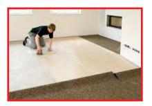
**4. INSTALLATION** - Adhering DAMTEC® acoustic underlay to substrate.
