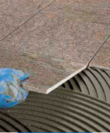
Installation of pre-glossed marble on floors
