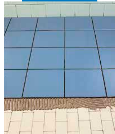
Tile on tile with Keraflex grey
