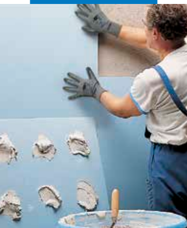
Fixing polystyrene foam slabs with Keraflex white
